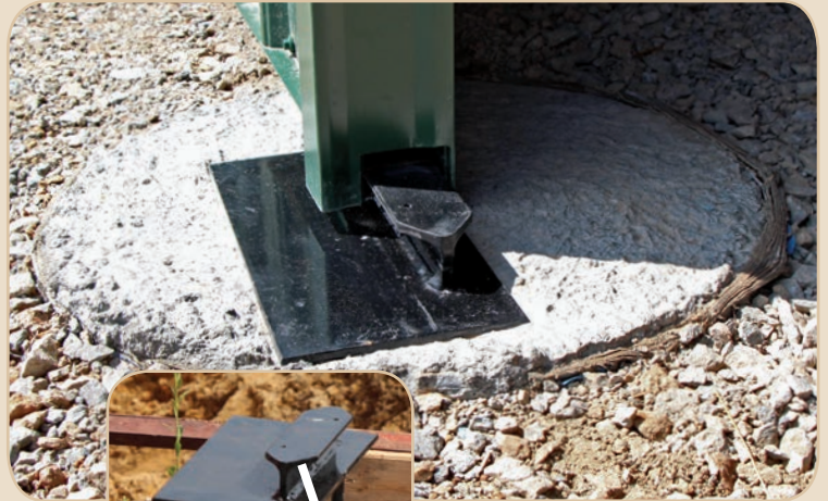
Concrete Center Door Stub
